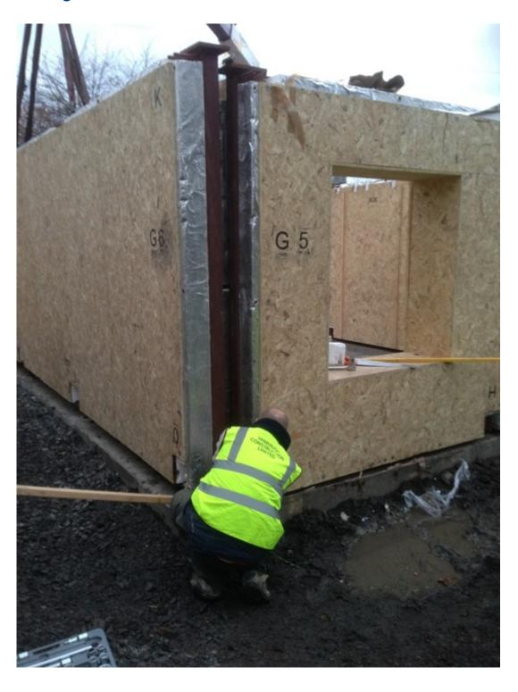
4. Erect the rest of the Wall Panels, bolting them to the Foundations, and Bolting them to the other Panels.
